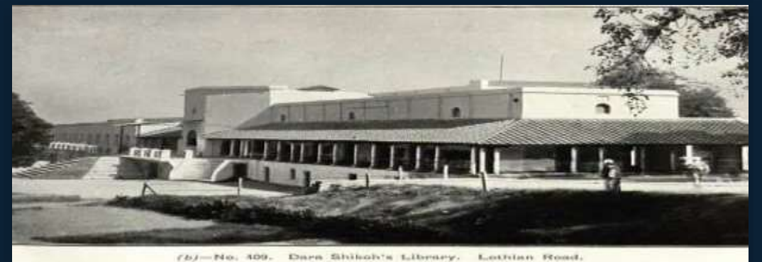
Dara Shikoh; his library in the 1850s; and the same building, remodelled, in a 1920s survey
